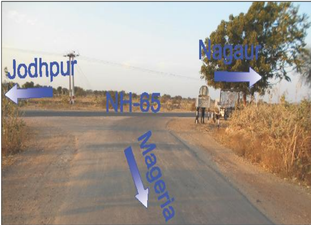
Figure 2.2: End Point (Khimsar, NH-65, Ch. 217.200)
